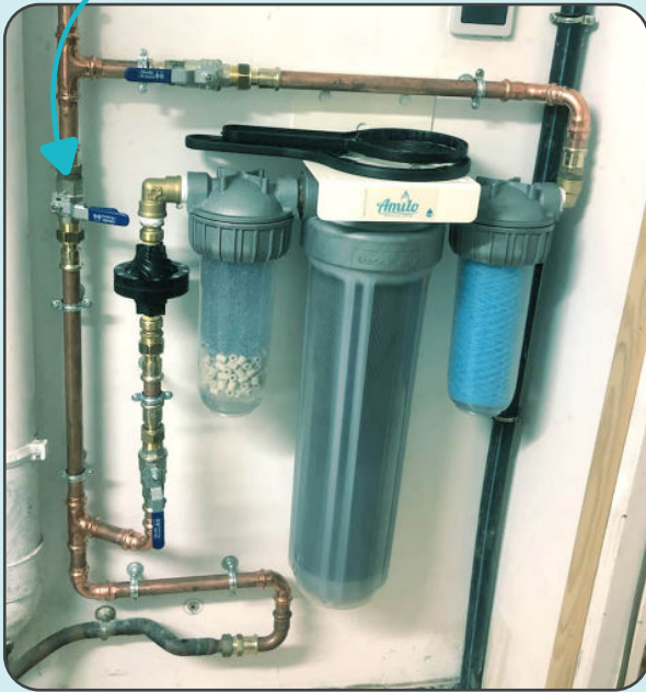
Vanne de bypass
